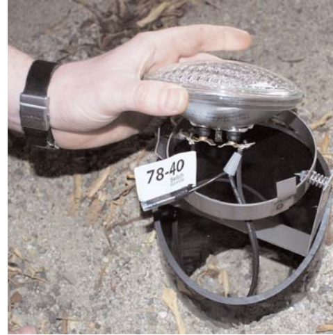
3. Remove lamp from gimbal ring.
