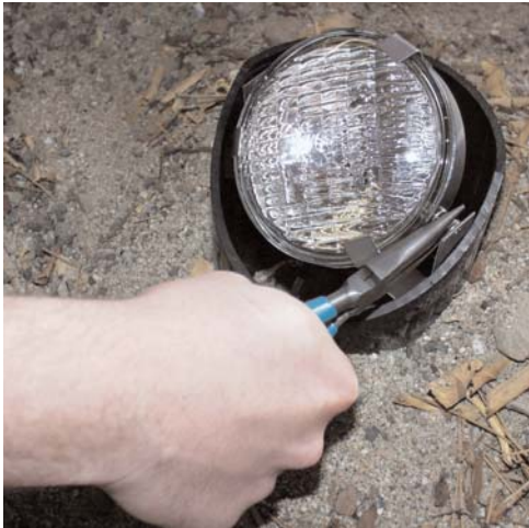
1. Remove gimbal ring & lamp from fixture body (needle-nose pliers recommended).
