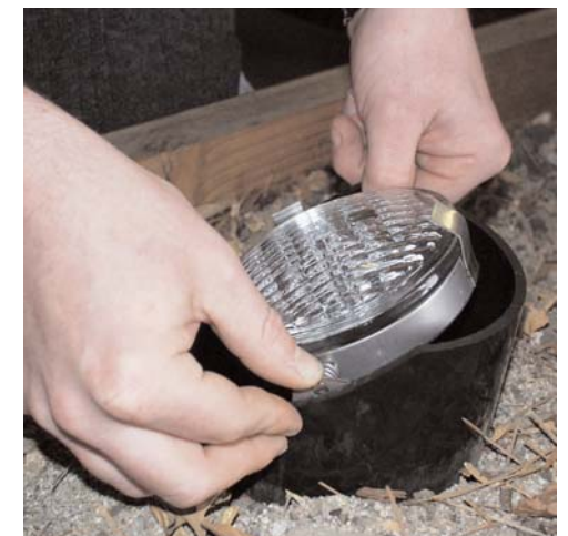
8. Replace gimbal ring and lamp back into casing.
