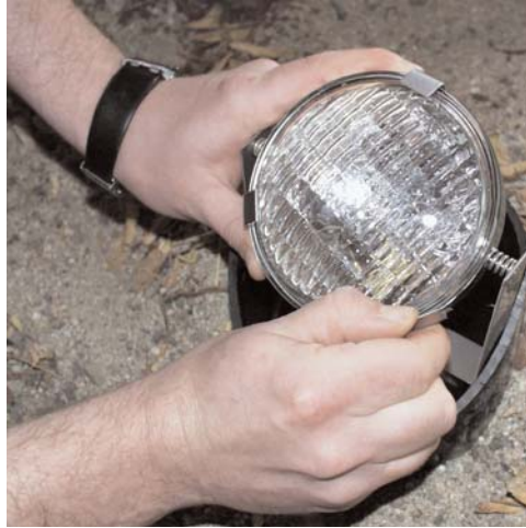
2. Bend back metal tabs securing lamp to gimbal ring.
