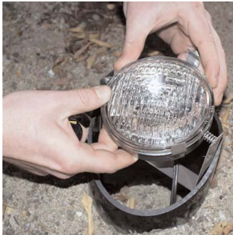
6. Place new lamp back into gimbal ring.
