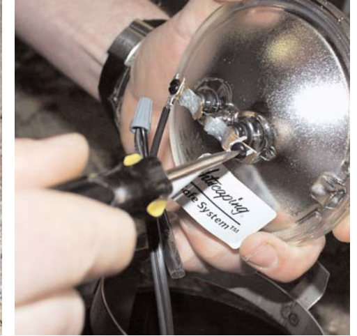
4. Disconnect lamp by loosening screw terminals.
